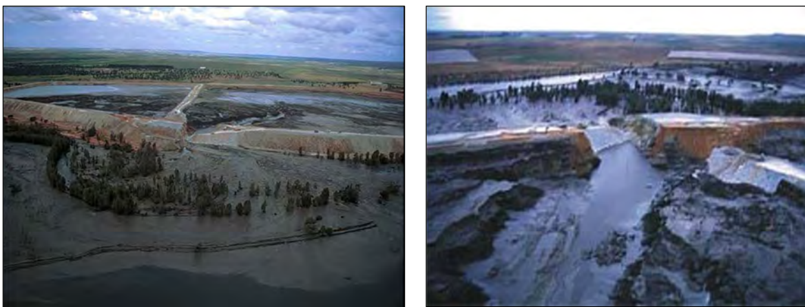
Fig. 3. Outpouring of slag as a result of tailings dam failure
